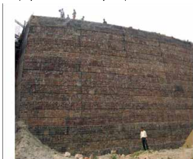
15 m high wall at Mayur Vihar End
