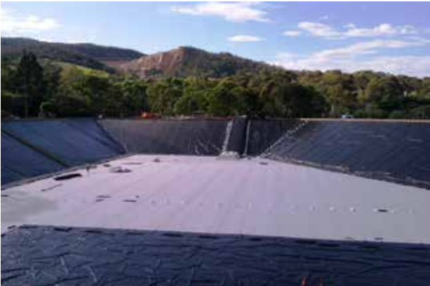
Cushion geotextile layer exposed during geomembrane installation
