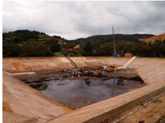
Removal of existing failed liner
