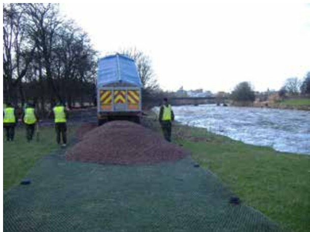
Base layer Tensar TriAx geogrid laid on the formation
