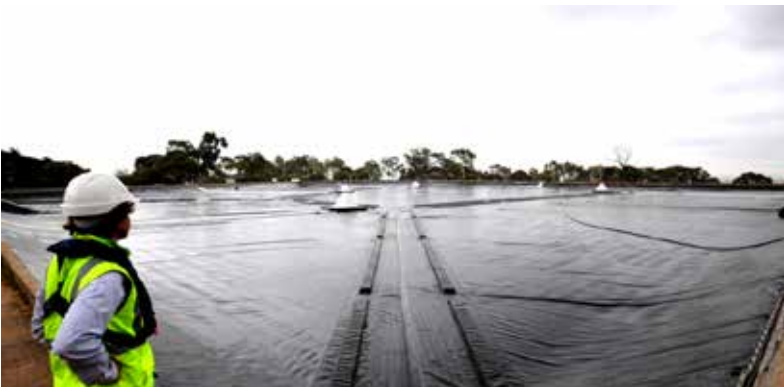
Cover installation complete
