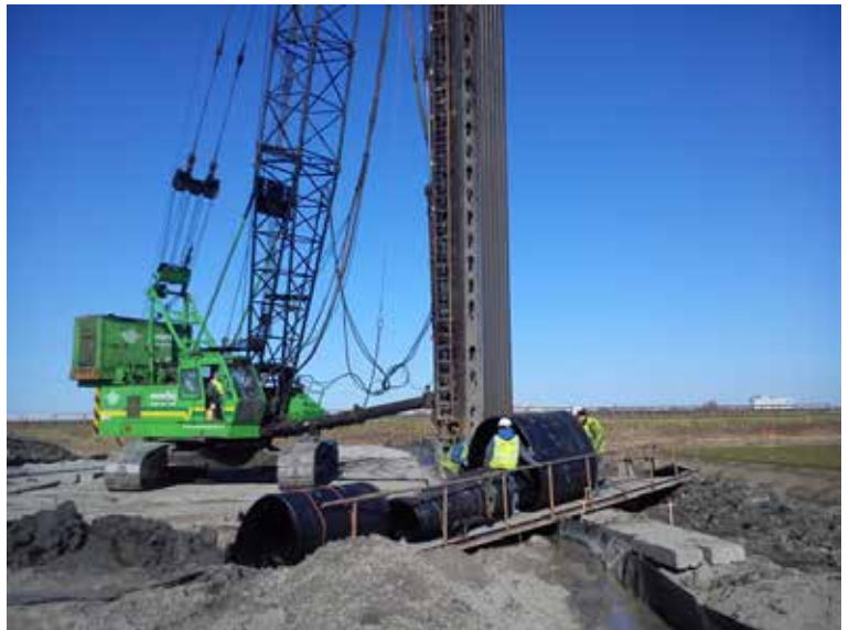
Photo 2 Installation of a membrane wall in Leeuwarden, Netherlands.
