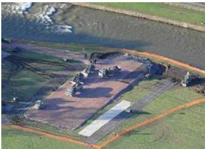
Aerial view of the temporary bridge span launching site
