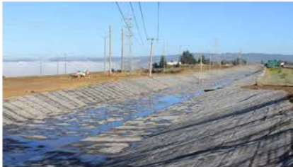
Morwell Main Drain rehabilitation - Australia -
