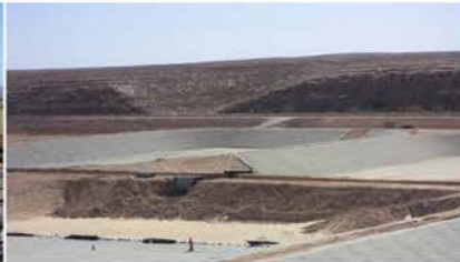
Gardhaia natural sewage treatment - Algeria -
