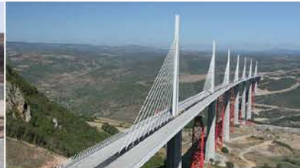
Millau Viaduct Bridge - France -
