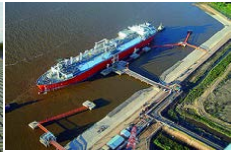
Completed work and operating dock
