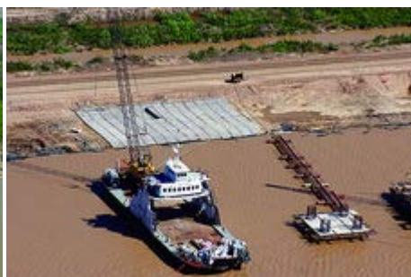
Precast blankets before installation
