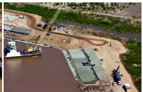
Installation of the precast blankets
