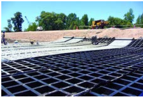
In – situ execution of the coating over the superior berm
