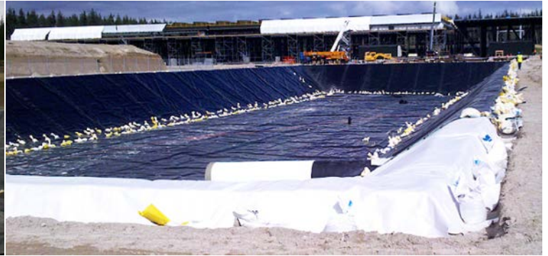
Lagoon during construction
