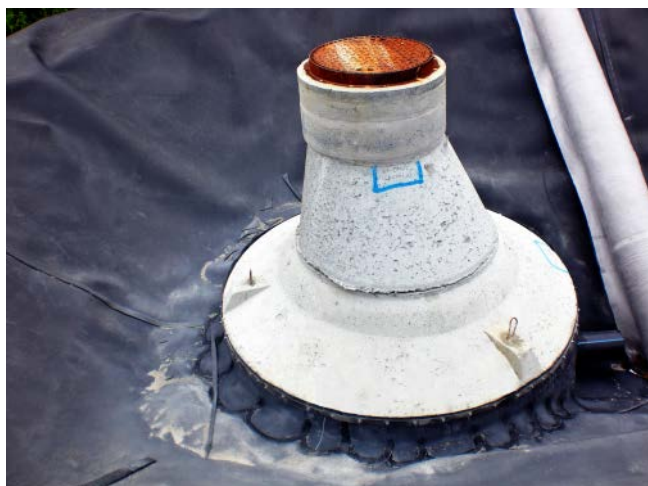
Integration of precast concrete shafts
