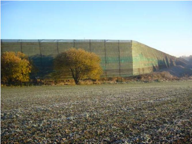
High reinforced soil structure with soft facing (lecture of V. Herle)
