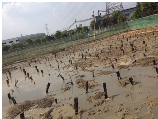
Fig.7 Soft ground before consolidation
