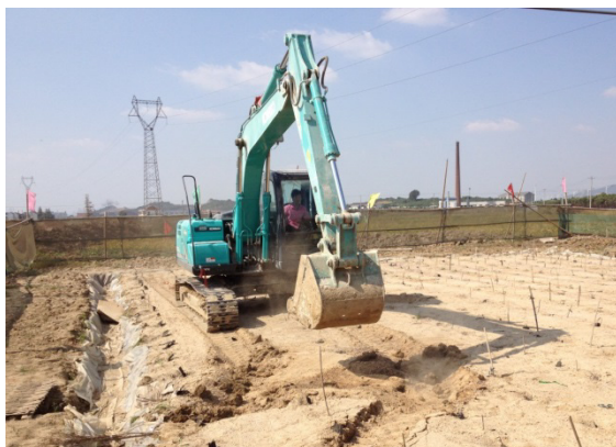
Fig.8 Soft ground after consolidation
