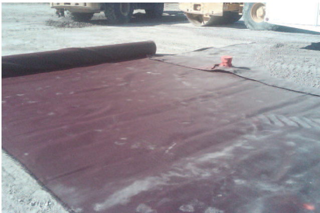
Mirafi® RS580i rolled out and overlapped appropriately
