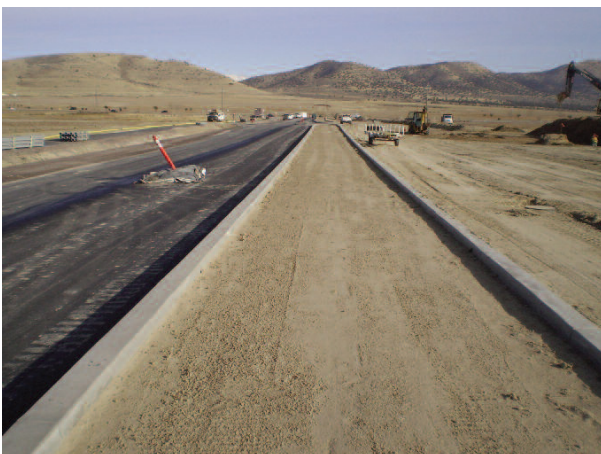
Phased construction - West lanes paved and open to construction traffic
