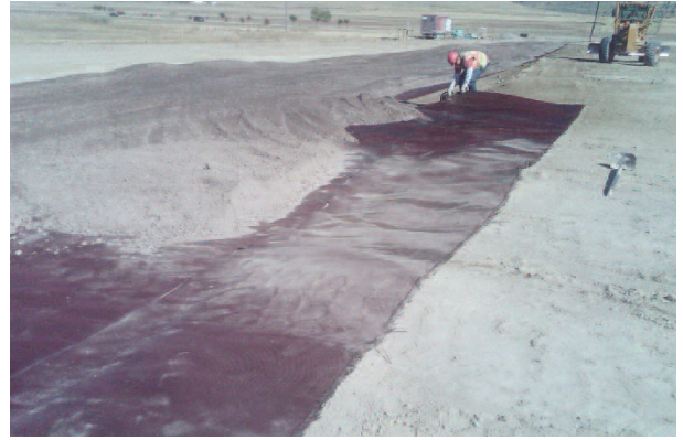
Base material being spread on Mirafi® RS580i
