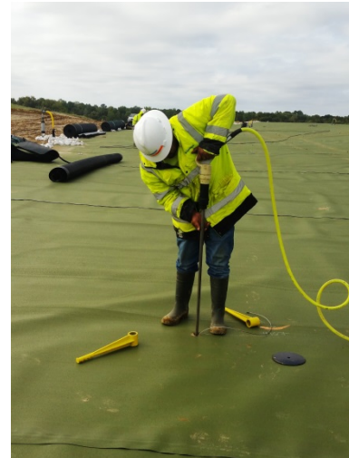
Anchor installation through the HDPE geomembrane with a light hydraulic breaker.
