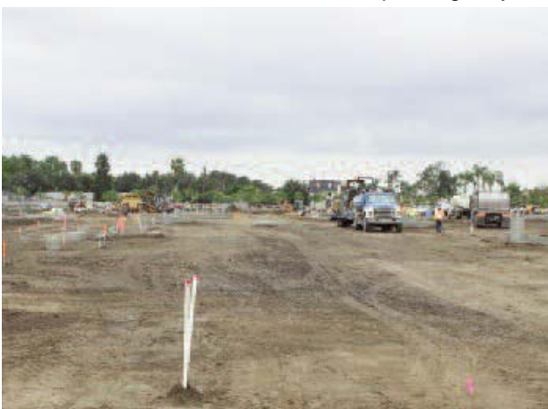
Project site native subgrade preparation
