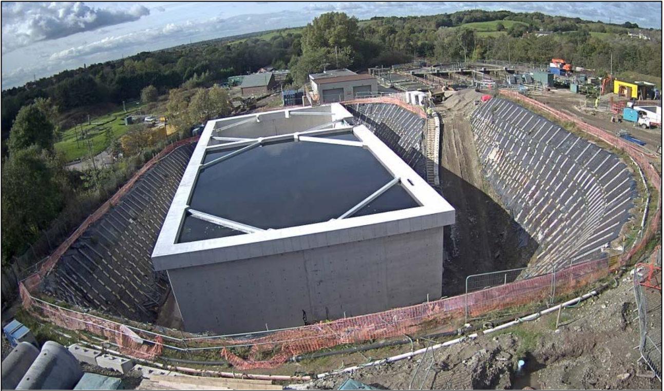
Completed temporary works with the retention tank in position
