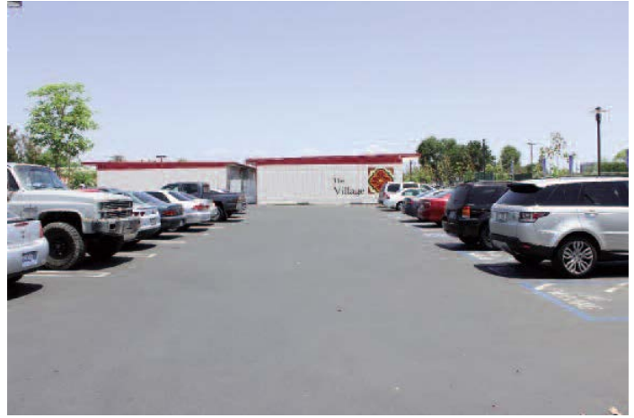
Completed asphalt parking area at Santa Ana College.
