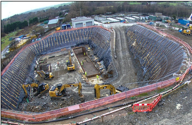
Slope reinforcement during excavation using Platipus anchors
