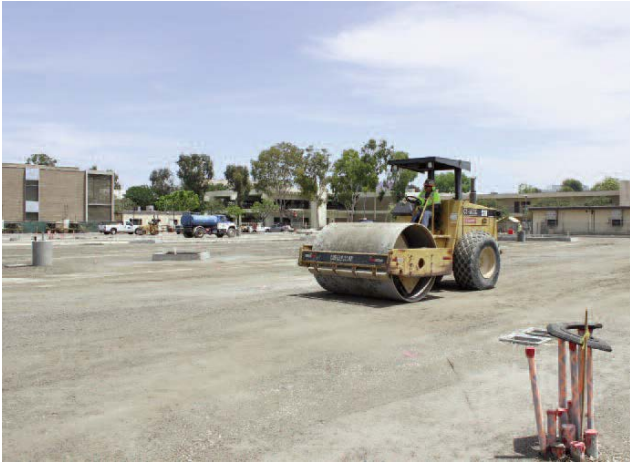
Compacting base material over Mirafi® RS380i
