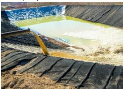
leads each day to the production of 24,000 m³ of washing and flotation sludge. This sludge contains between 70 and 80% of water, 80 to 85% of this water is recovered from the decanters and the remainder is evacuated as thickened sludge to ponds. OCP wanted to cover the traditional pond with a solution to increase the water removal from sludge and preserving the slopes of ponds from the soil erosion. This request also comes within the framework of the COP 22 which took place in Morocco in 2016.
