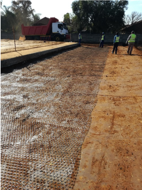
Installation of first row complete
