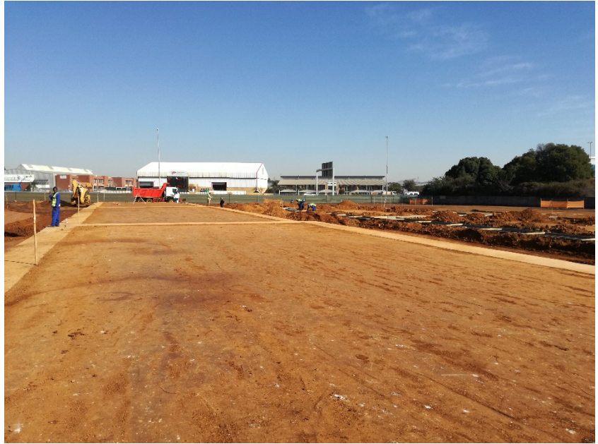
Platforms which will function as base for shipping containers
