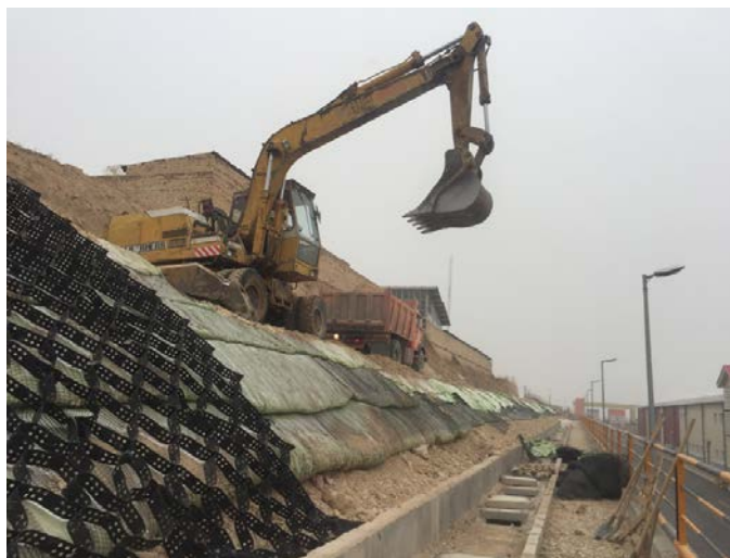
Different Geosynthetics layers in a green reinforced slope
