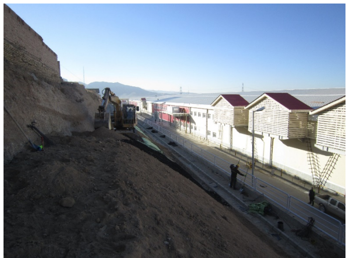
General View of The project
