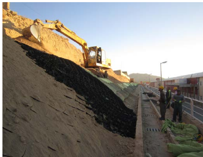
Covering the slope with vegetative soil
