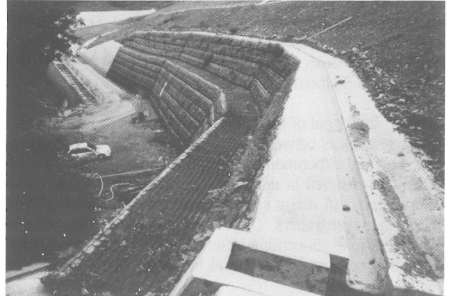
Slope Stabilization Using Geogrids
