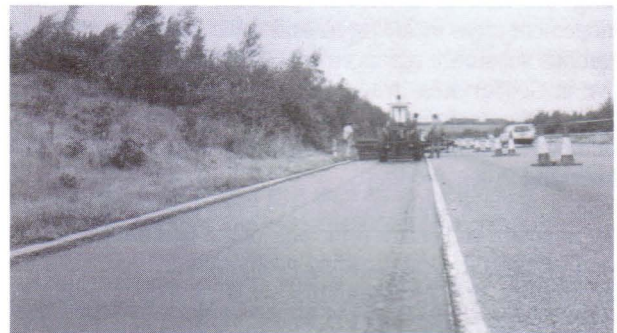
Polyfelt PGM laid mechanically into the previously applied bituminous tack coat
