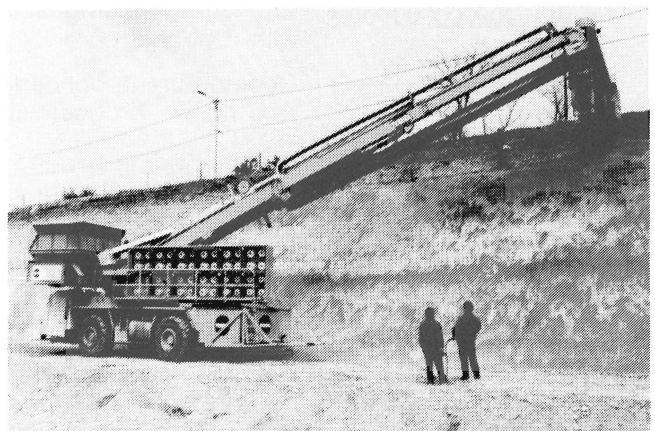
Texsol wall under construction
