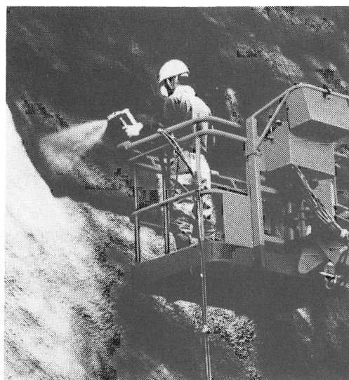
Spraying of S.B.R. - asphalt emulsion
