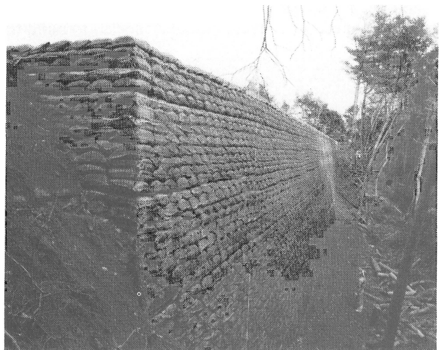
Example of a steepened slope using NESTEM geogrid
