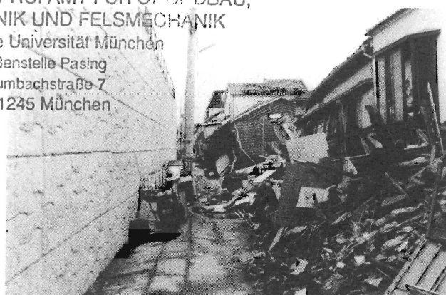
Failure of a conventional railway support wall.
