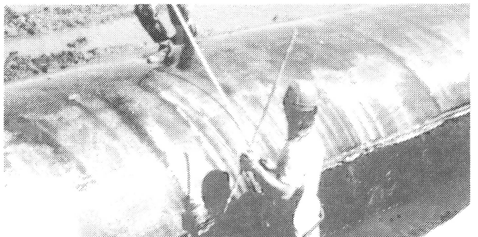
Figure 2. Geometry of tube filled with clayey slurry immediately after completion of pumping.
