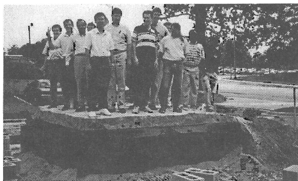
Professors on the demonstration modular block wall.
