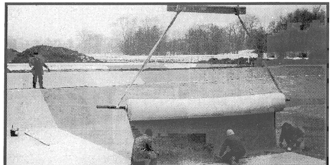
Installing a large area of Geofelt Bentonite Liner (GBL).
