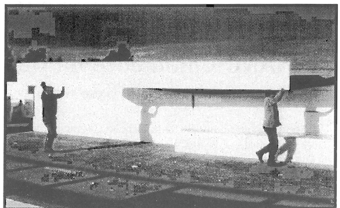
Figure 2. Workers carrying large block of geofoam.
