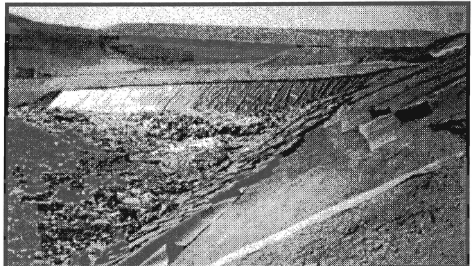
Slide in a municipal waste landfill.
