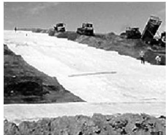
Bentomat ST GCL used at the defunct Gary, Indiana, USA landfill.
