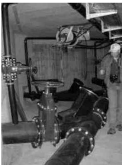
Aurach Landfill (Germany): in the horizontal shaft.
