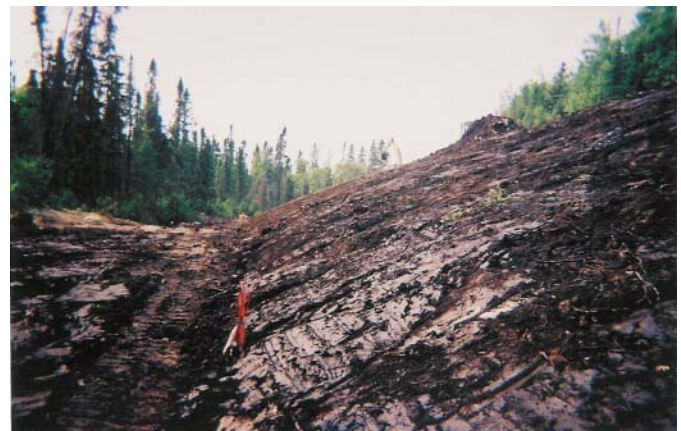
Figure 2. A 9-m high railway embankment extension was constructed on a soil clay deposit within a tight schedule by accelerating consolidation and strength gain using PVDs.
