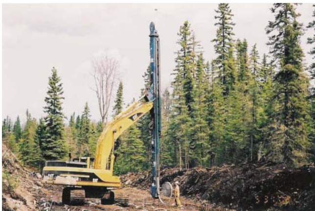
Figure 2. A 9-m high railway embankment extension was constructed on a soil clay deposit within a tight schedule by accelerating consolidation and strength gain using PVDs.
