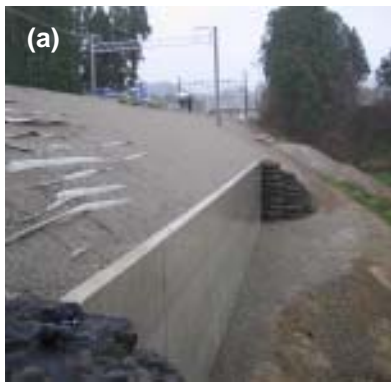
Figure 4. Reconstructed geogrid-reinforced soil (GRS) retaining wall at Site 1 with a full-height rigid facing built using the staged construction method: (a) 5 December 2004, photo taken by F. Tatsuoka; and (b) the first train running on the wall, 26 December 2004 (photo is courtesy of East Japan Railway Company).
