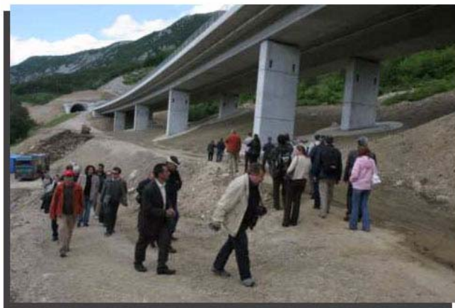
Technical visit to the motorway construction site near Postojna.
