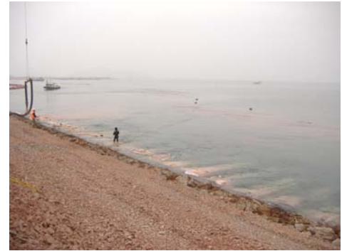
Figure 2. Geotextile tube mattress filter (SMG Sea Dyke).
