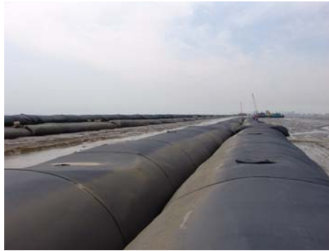
Figure 1. Temporary construction platform (Incheon Grand Bridge).
