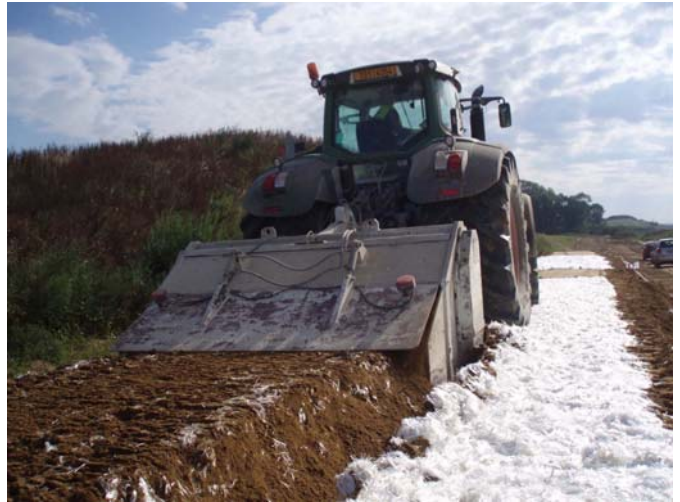
Mixing PET fibres into the soil (lecture of H. Rubisarova)
