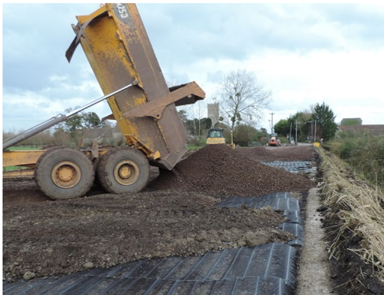
Tensar stabilised causeway nears completion
